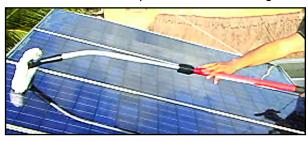
8) Mop the surface of the panel using back and forth or side to side motions. You can either allow the panel to air dry, or squeegee the excess water off of the surface.
