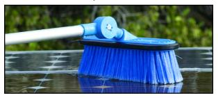
6) Start by rinsing the surface of the panel, then with the brush, apply light pressure using a scrubbing motion.
